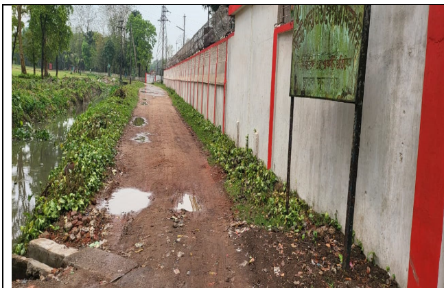
Road for rehabilitation: Chhatak Poursava
